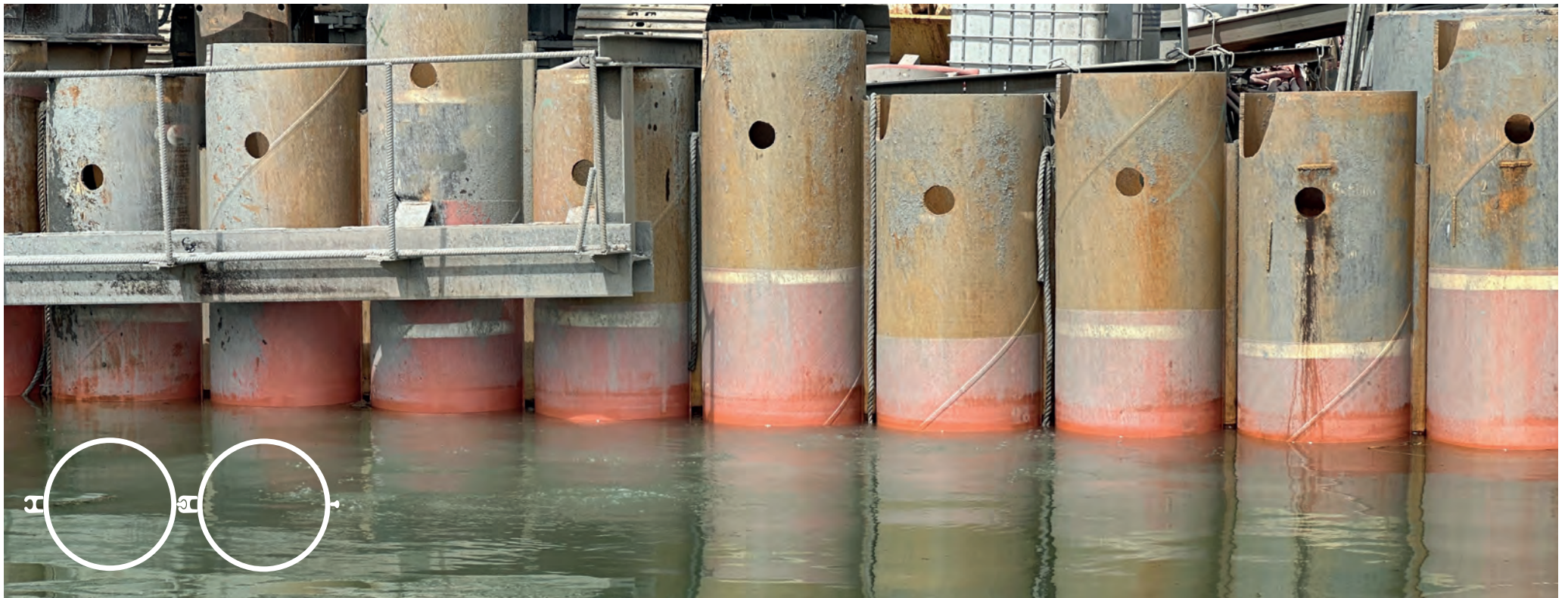
MF-Pipe - Vibro-/Impact driving with SteelWall connectors
