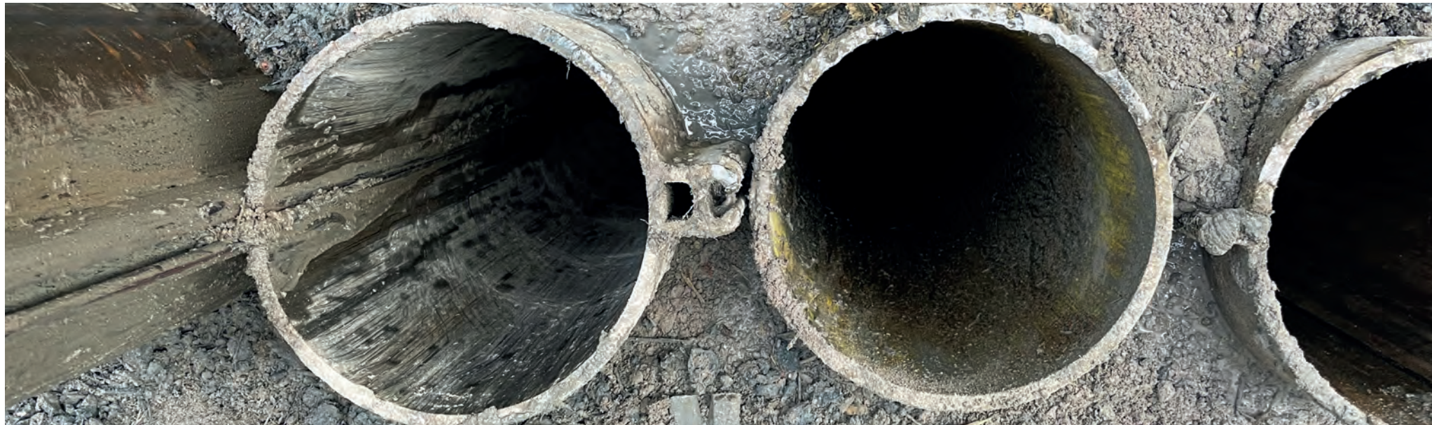
MF-Pipe - DTH procedure with SteelWall connectors
